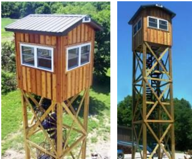
Figure 1-64. Lookout for observing nature, hunting and outdoor recreation. Stands 30 ft. from ground to floor, and 41 ft. to the peak of the roof. The building features 44-ft. long foundation-grade treated four-ply laminated columns on 4 ft. deep embedded footings.
