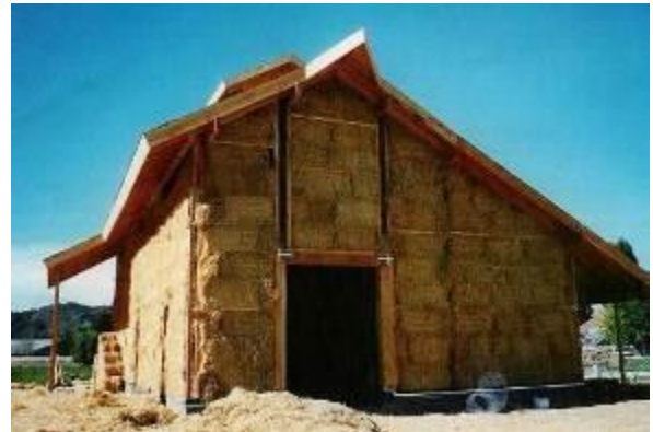
Figure 1-56. Non-structural straw bale walls prior to plastering. Image from the American Society of Agricultural and Biological Engineers. Used with permission.
