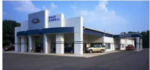
Figure 1-36. Commercial post-frame building clad in stone and smooth metal panels. An FBi Buildings project.
