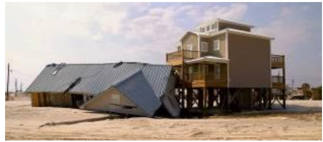
Figure 1-60. Sound engineering and construction of this post-frame stilt building on Dauphin Island, Alabama saved it from meeting the same fate as the one deposited in its front yard by Hurricane Katrina. FEMA photo.
