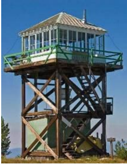
Figure 1-63. Forest fire lookout towers are great examples of how post-frame construction can be used to frame towers. Shown here is the Granite Mountain Lookout, Alpine Lakes Wilderness Area, Washington.
