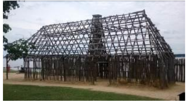
Figure 1-28. Frame of pole building barrack erected in 2011 in an effort to duplicate construction methods used during the colonization of Jamestown. Located behind the replicate barrack is a replicate palisade.
