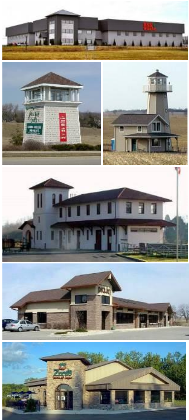
Figure 1-65. Tower applications are ideal for post-frame. An FBI Buildings project.
