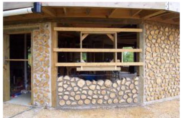
Figure 1-57. Cordwood (a.k.a. stackwood) infill walls.
