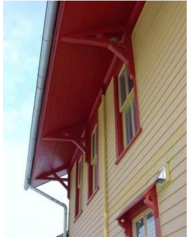
Figure 1-75. Wall support brackets used to support a roof overhang.
