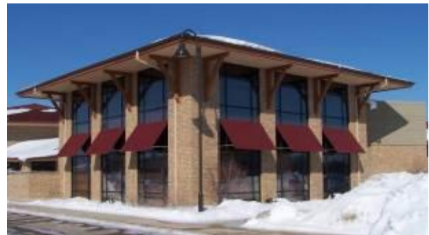
Figure 1-76. Tall walls, large regularly-spaced windows and wall brackets make buildings similar to this good candidates for post-frame.
