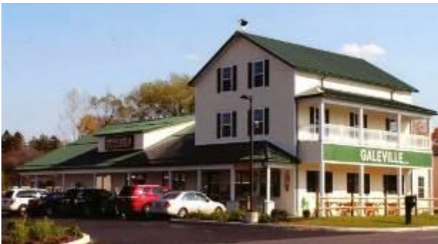
Figure 1-66. Post-frame convenience store for Byrne Dairy in Galeville, NY. The storefront features a porch and above balcony. A porch formed by a roof overhang extends along the side of the structure.
