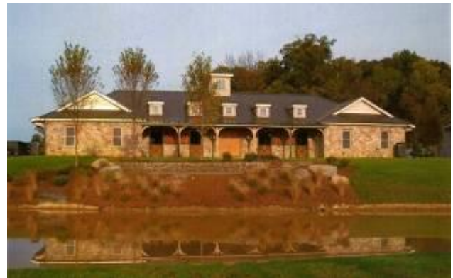
Figure 1-68. Post-frame horse barn with post-supported roof overhang.
