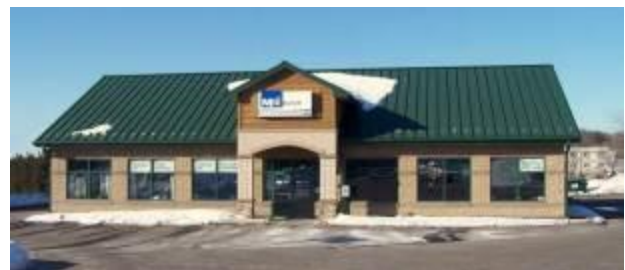
Figure 1-40. Large, equally spaced windows suit post-frame.
