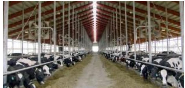
Figure 1-44. This building is typical of many dairy freestall barns. The greater width of these buildings results in (1) tall gable endwalls requiring substantial framing, and (2) the need for interior support posts.
