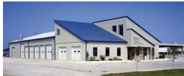
Figure 1-39. Post frame readily accommodates the overhead doors required for this automobile repair business in Lafayette, Indiana. An FBi Buildings project.
