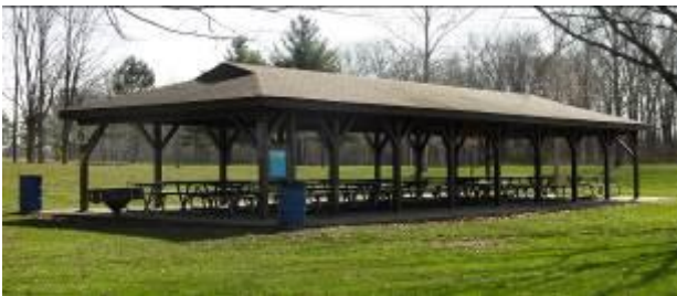
Figure 1-46. The desire for open sidewalls makes the post-frame building system a popular choice for park and other recreational shelters.
