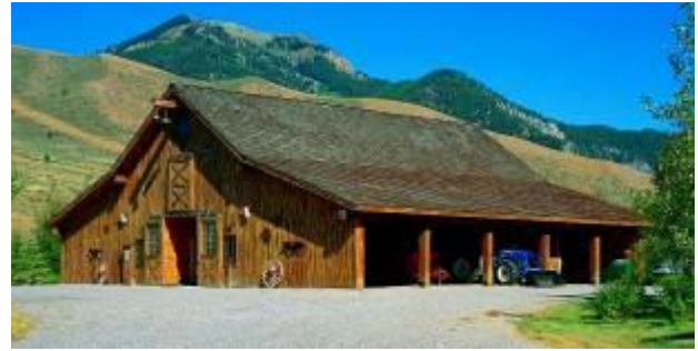
Figure 1-48. Open front equipment storage building.
