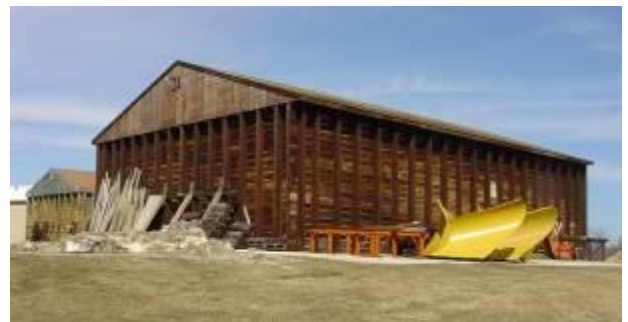
Figure 1-45. High wall pressures and resistance of wood to corrosion make post-frame the perfect application for salt storage facilities.
