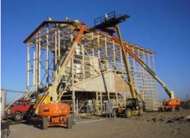
Figure 1-42. Post-frame concrete batch plant with a 45 ft ceiling height, accomplished in part by bracing wood columns back to the main structure of the concrete plant equipment.
