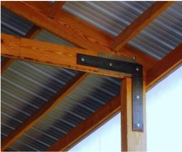
Figure 1-54. Truss resting on outer ply of a laminated post. Steel L-bracket placed on outer face of truss to help reinforce post-to-truss connection.
