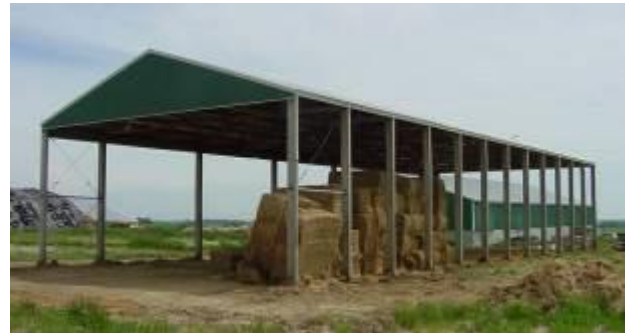
Figure 1-49. Hay storage facility with all-around access by. Post spacing on back endwall twice that on front endwall to accommodate machinery access.
