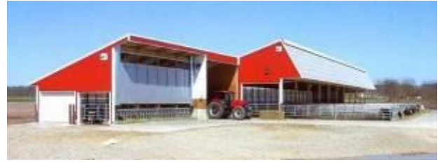
Figure 1-47. Heifer growing facility with open sidewalls.
