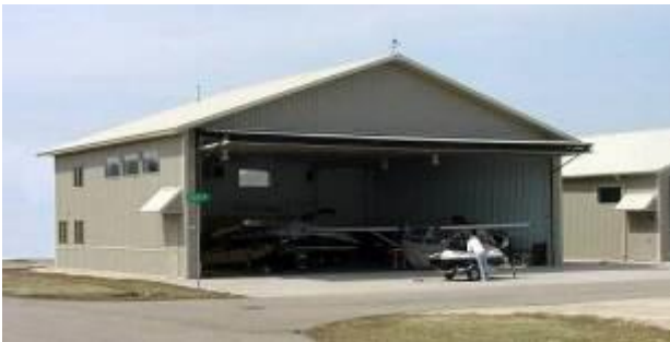
Figure 1-43. The ability to construct inexpensive buildings with relatively high eave heights makes post-frame ideal for many machinery storage buildings including this airplane hanger.
