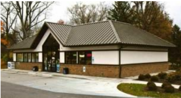
Figure 1-34. Small commercial post-frame building sided with stucco and brick veneer.
