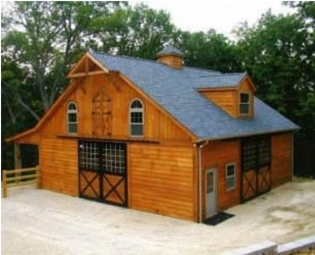
Figure 1-33. Wood-clad post-frame building constructed for horse housing.
