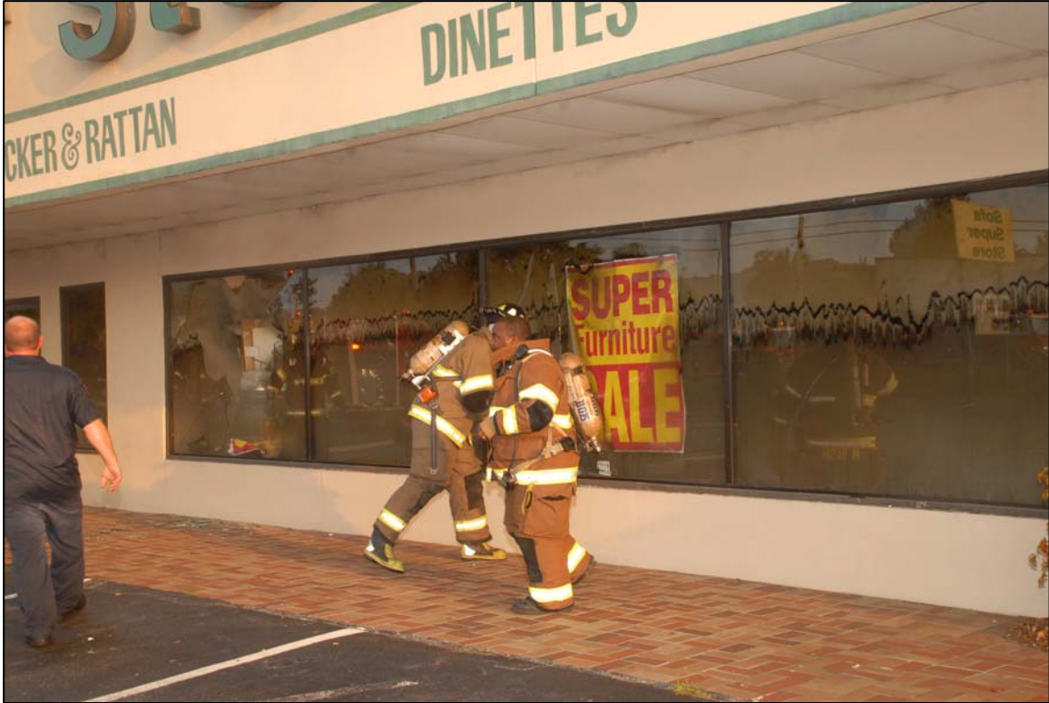
Photo 6: Firefighters break out windows to the right of the store entrance. Note air being drawn into the broken windows to the left of the firefighters. The heat stratification inside the showroom is evident. This photograph was taken at 19:35:31. (Photo courtesy of Bill Murton, Charleston Police Department)
