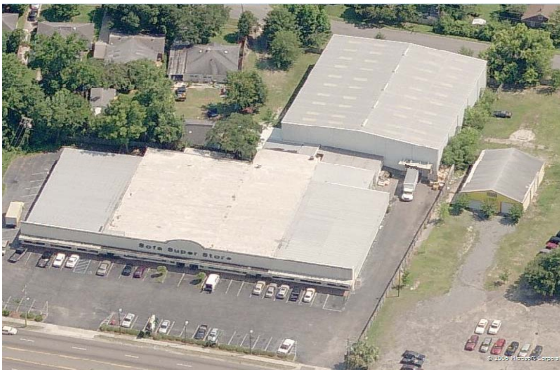
Photo 1: Aerial view of the north side of the Sofa Super Store. (Photo courtesy of Pictometry, International)
