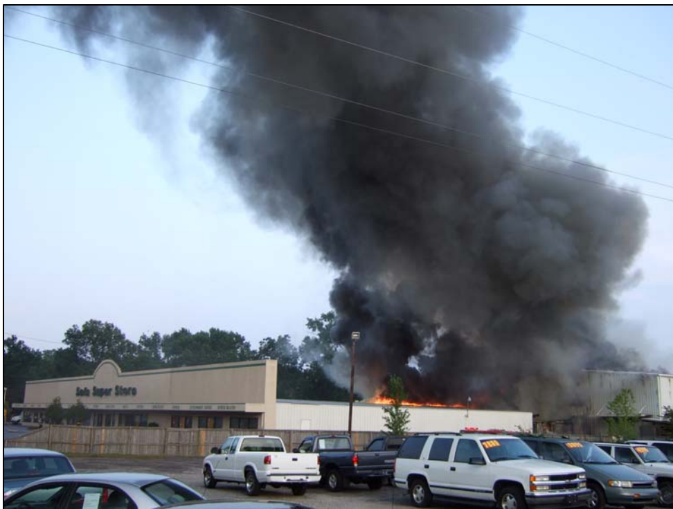
Photo 9: Fire visible from the roof of the retail area. This photo was taken at 19:23:16. (Photo courtesy of Dan Folk)
